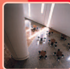
Joints de dilatation
