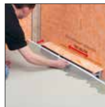
=> 4. Ajuster le support de caniveau
