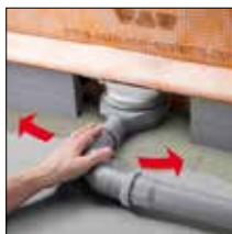
=> 5. Ajuster le tuyau d'évacuation
