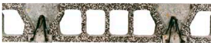
Dalle de compression coulée in situ
